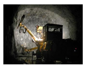
Initially a smaller 5 x 6m relief tunnel was conventionally blasted in the top middle section of the larger tunnel excavation.
